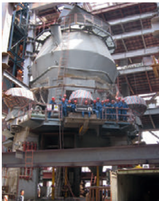
Loesche mill Type LM 56.3+3 CS, under construction, Ras al Khaimah, United Arab Emirates, 2007
