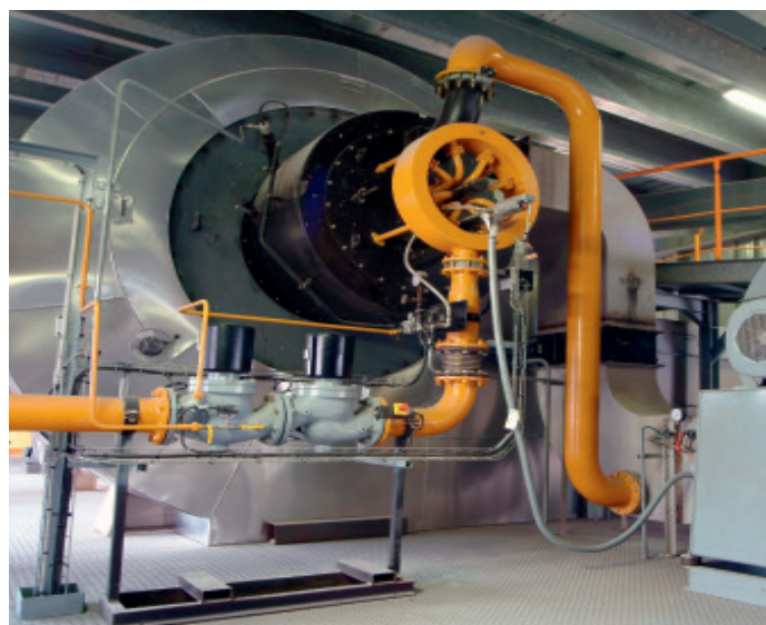
LOMA combustion unit type LF 25 with a natural gas burner in the central grinding plant for granulated blast furnace slag, Dunkerque, France, 2005
